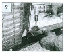
Install the side opening grille inserts. Install a screw from the front; secure a J hook and nut onto each screw. Center one of the inserts; Wrap the J hooks around the inner cross bar mesh. Tighten the hardware.
