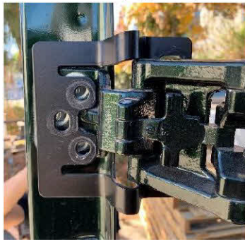
Figure 3: Bracket Installed Over Factory Hinge
