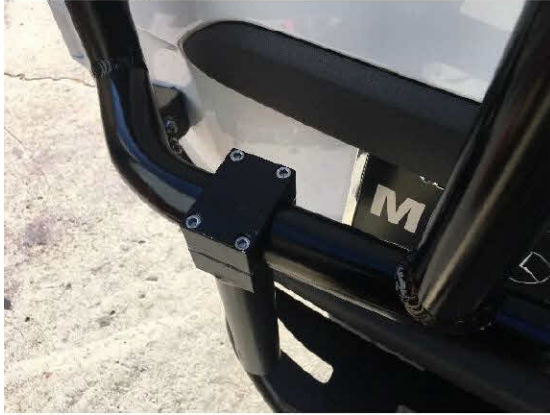
Figure 1: Bolt-On Supports Loosely Bolted to Lower Crossmember
