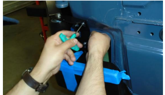
Figure 12: Tightening Hardware Through Insert Opening
