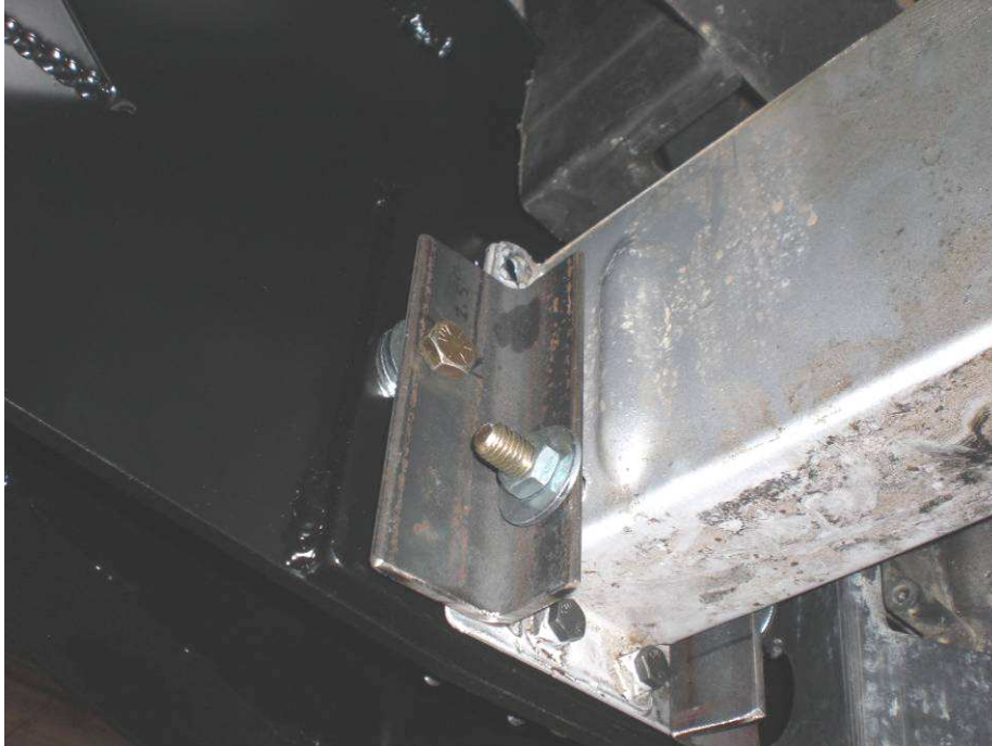
Figure 11: Steel support brackets bolted to frame
