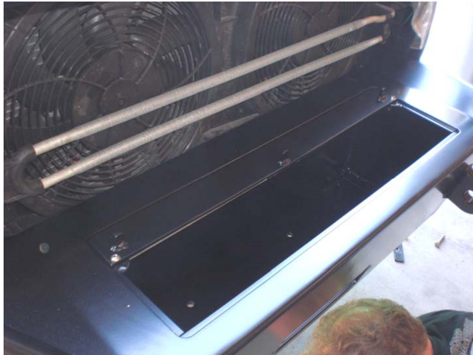
Figure 12: Bumper door, rear portion installed
