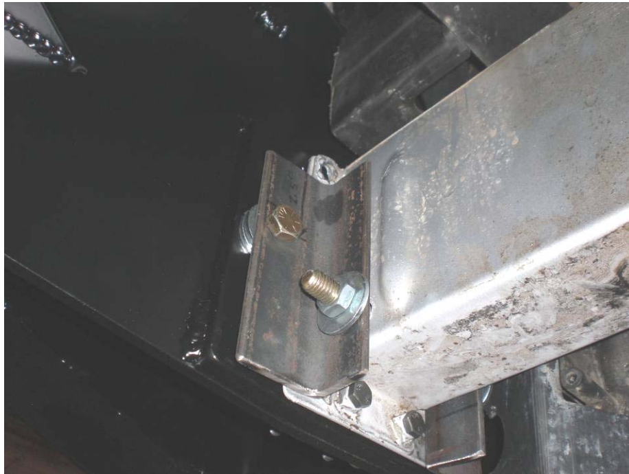
Figure 11: Steel support brackets bolted to frame
