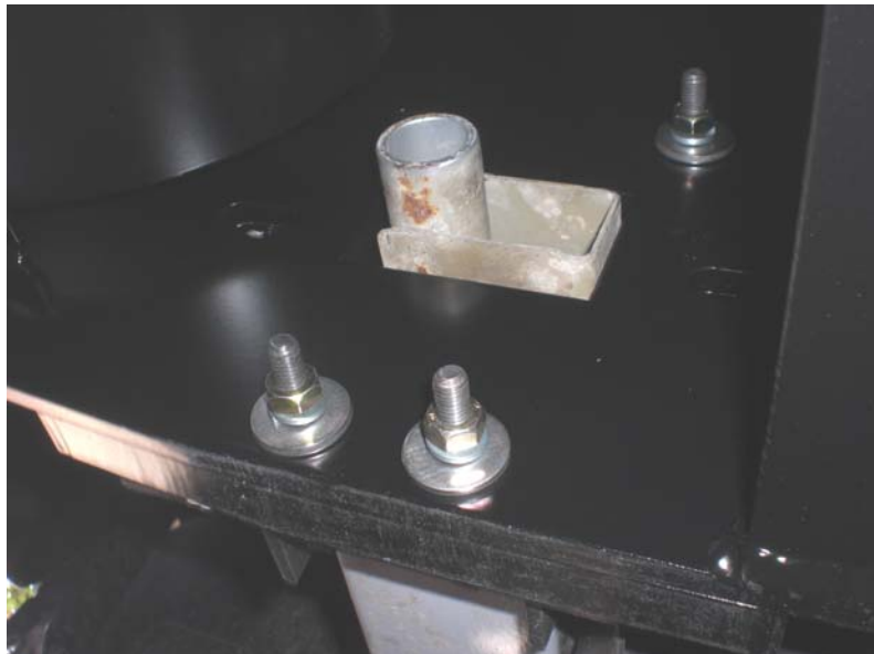
Figure 9: Frame mounting bolts with lock washers and 3/8" washers installed
