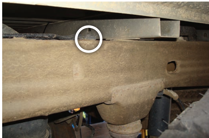
Outside frame, left hand (driver side) view
