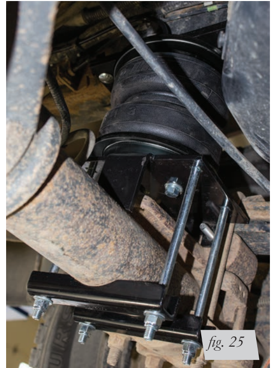
Left side (driver): front view of installation.
