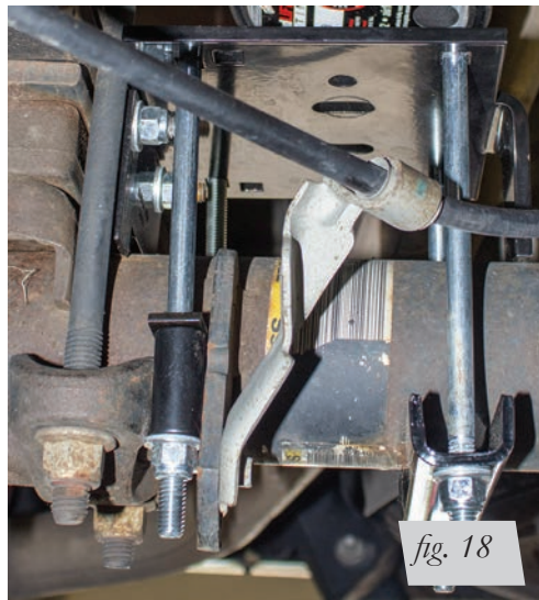
Right side (passenger) forward axle view of finished installation torqued to 10 lb.-ft.
