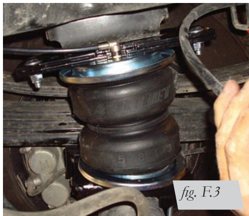
Inside view of the driver's side installation.
