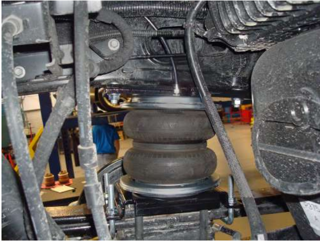
Inside view of driver's (left) side installation. Fig. 24
