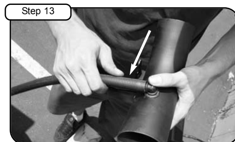
Step 13 Install 1/2" hose on fitting.
