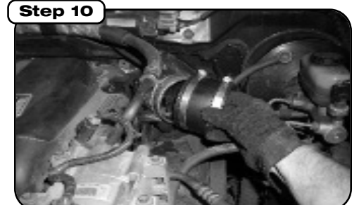
Place provided clamps loosely over provided coupler and place onto factory turbo inlet elbow
