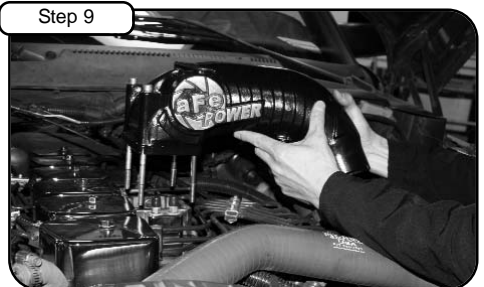
Step 9 Carefully install aFe manifold into vehicle. Guide screws through gaskets and air grid heater.
