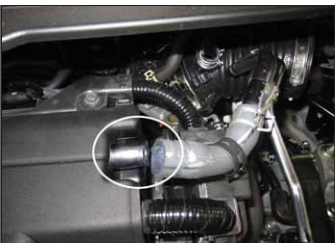
s. Release the clip on the valve cover for the PCV hose, then remove the hose from the valve cover.
