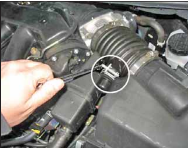
g. Loosen the clamp securing the positive crank case ventilation (PCV) resonator.
