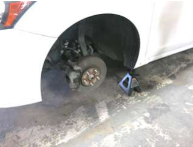
g. Jack up and support vehicle safely with jack stands. Remove the driver side wheel and pull inner fender to access intake resonator for removal by removing the 10mm push clips.
