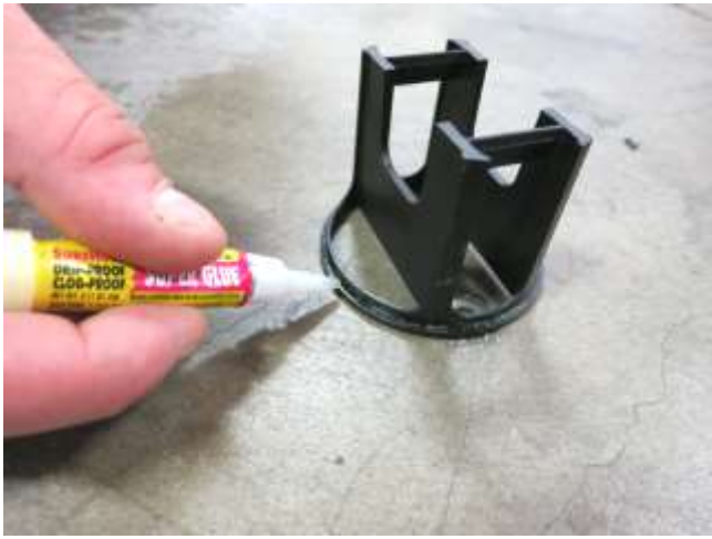
f. Apply the included super glue to the plastic air straightener as shown.
