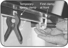
B. Hold rail in place with spring clamp and close tailgate to check height. Then place 1st clamp as close to front as possible and use a 1/2" wrench to tighten.
